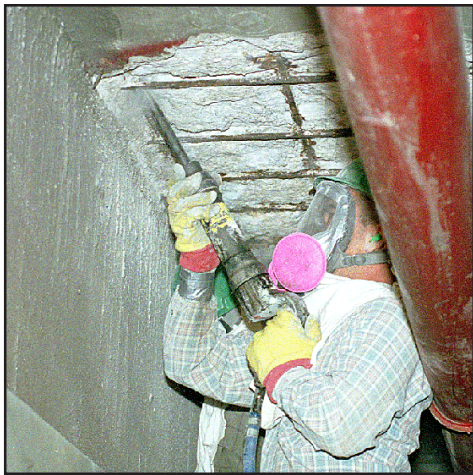
Western craftsman removes deteriorated concrete
